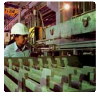
Top: Switchyard of 540 MW CPP at BALCO.
